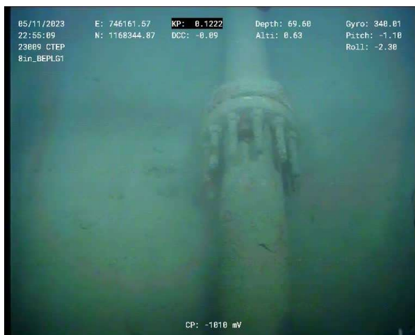
Figure 9 – BEWG Sealine Tie-in Flange KP 0.122 (Top View)
