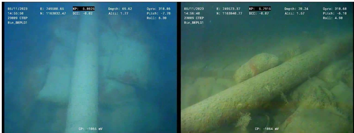
Figure 29 – 12" BEPLB2 pipeline Crossing under 8" BEPLG1 at KP 5.803 (View from top)
