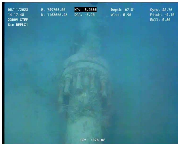
Figure 21 – BEWA Spool Tie-in Flange KP 6.036 (Top View)
