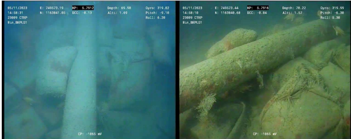
Figure 31 – 12" BEPLB1 pipeline Crossing under 8" BEPLG1 at KP 5.792 (View from south east)
