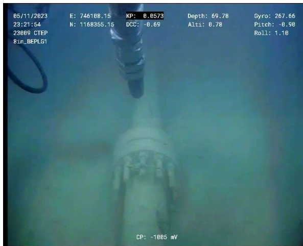
Figure 5 – BEWG Spool Tie-in Flange KP 0.057 (Top View)
