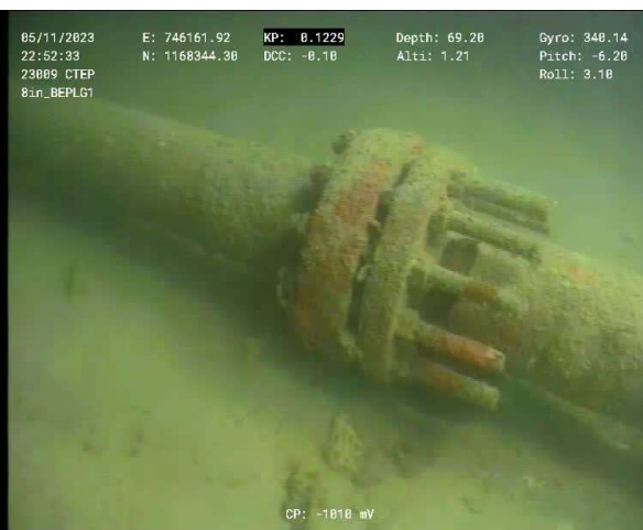
Figure 10 – BEWG Sealine Tie-in Flange KP 0.122 (Side View)
