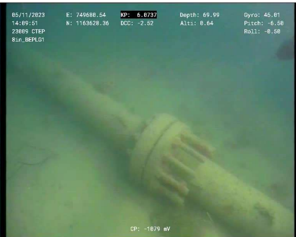
Figure 20 – BEWA Spool Tie-in Flange KP 6.073 (Side View)
