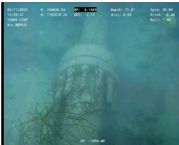
Figure 15 – BEWA Spool Tie-in Flange KP 6.147 (Top View)
