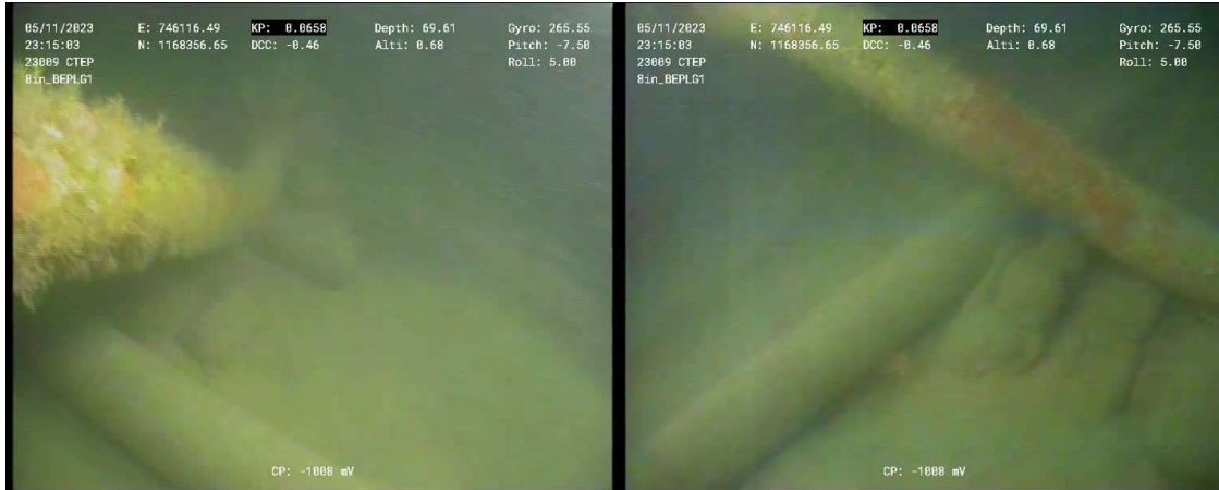
Figure 35 – 6" BEWLG Crossing Over 8" BEPLG1 at KP 0.063 (View from south)
