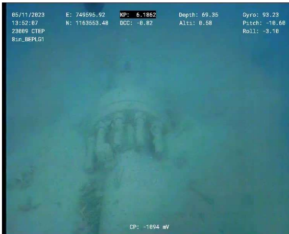
Figure 13 – BEWA Spool Tie-in Flange KP 6.186 (Top View)
