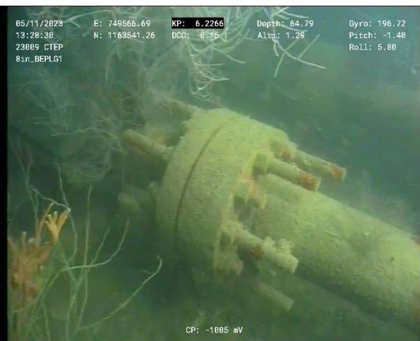
Figure 12 – BEWA Riser Tie-in Flange KP 6.227 (Side View)
