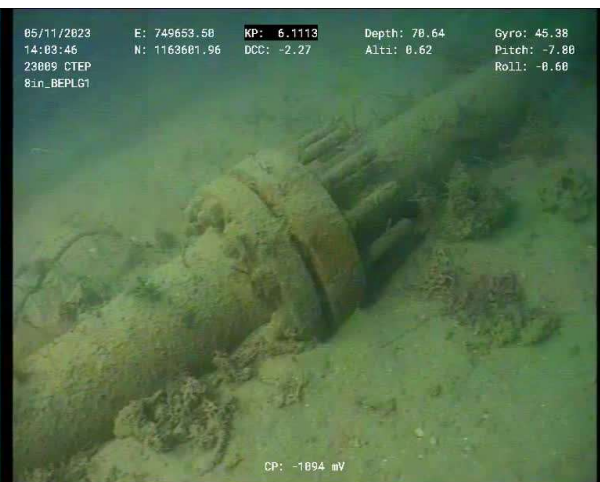
Figure 18 – BEWA Spool Tie-in Flange KP 6.110 (Side View)
