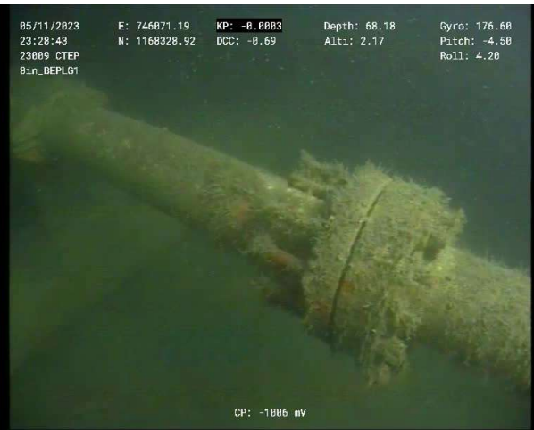
Figure 4 – BEWG Riser Tie-in Flange KP -0.001 (Side View)
