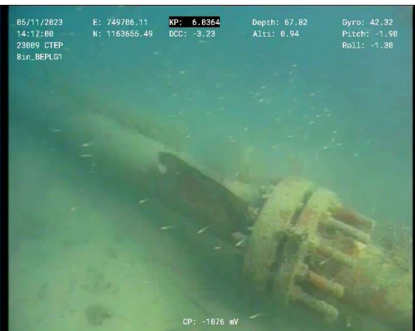
Figure 22 – BEWA Spool Tie-in Flange KP 6.036 (Side View)
