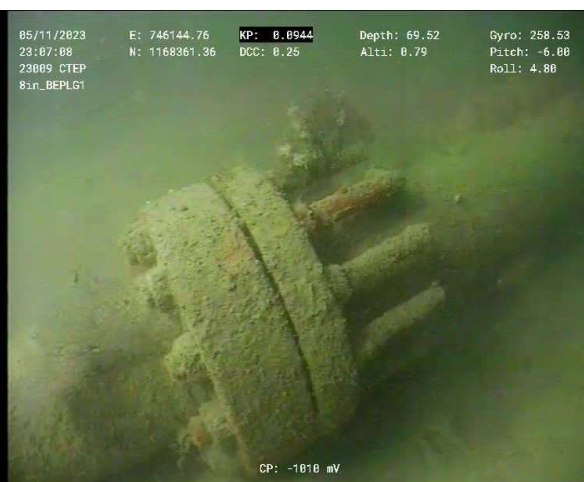
Figure 8 – BEWG Spool Tie-in Flange KP 0.094 (Top View)
