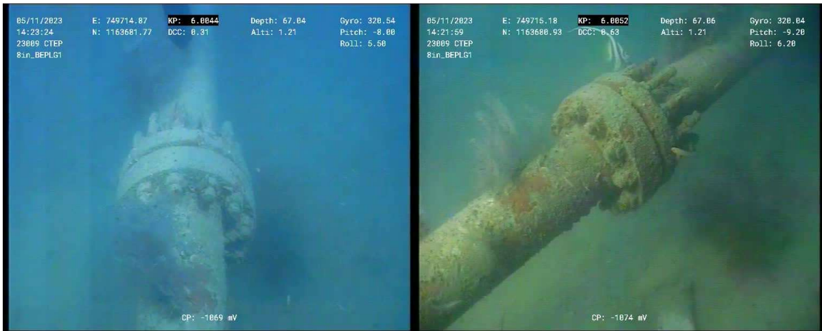
Figure 23 – BEWA Sealine Tie-in Flange KP 6.004 (Top View)
