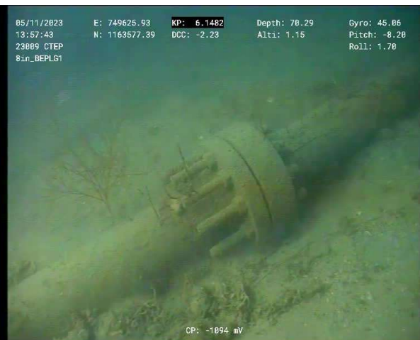
Figure 16 – BEWA Spool Tie-in Flange KP 6.147 (Side View)
