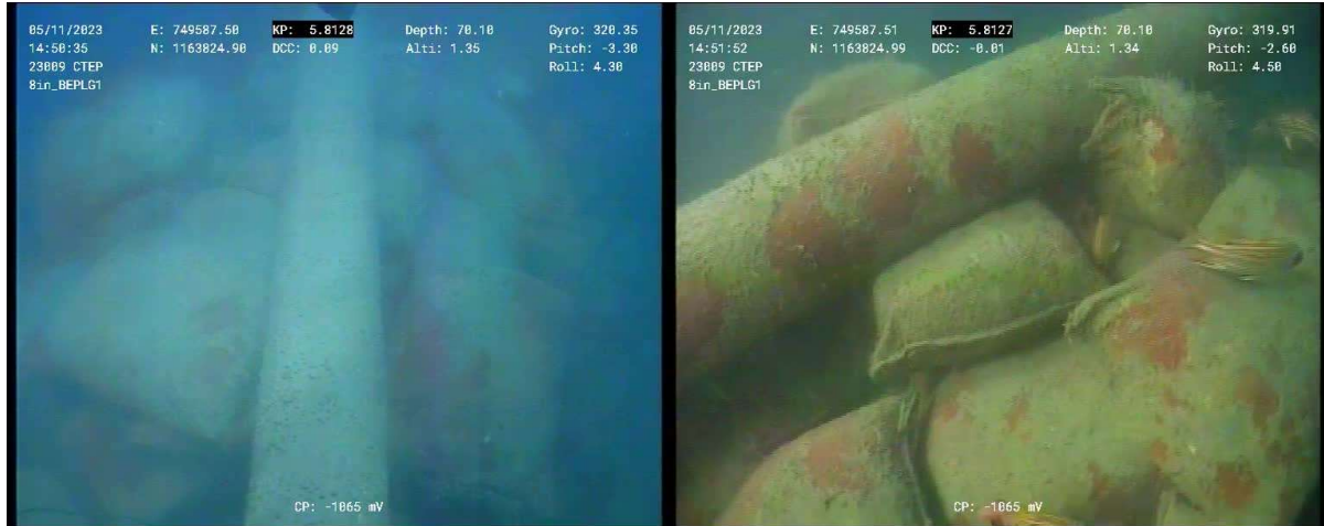
Figure 27 – 12" BEPLB2 pipeline Crossing under 8" BEPLG1 at KP 5.813 (View from top)
