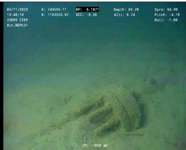
Figure 14 – BEWA Spool Tie-in Flange KP 6.186 (Side View)
