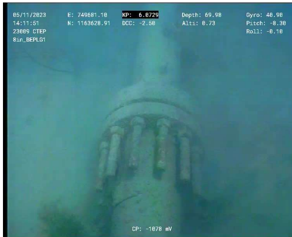
Figure 19 – BEWA Spool Tie-in Flange KP 6.073 (Top View)
