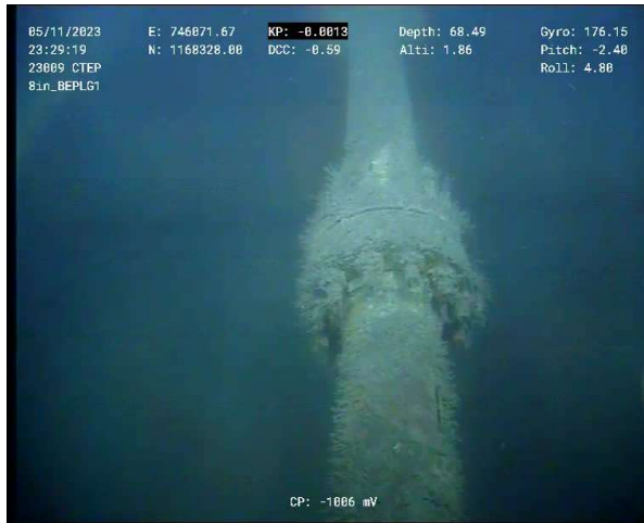
Figure 3 – BEWG Riser Tie-in Flange KP -0.001 (Top View)
